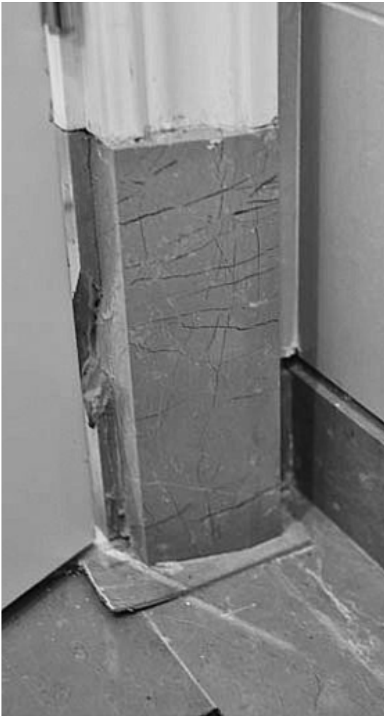
墙柱有破损
